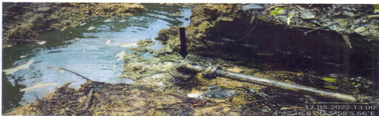
SPILL POINT AFTER ECAVATION
