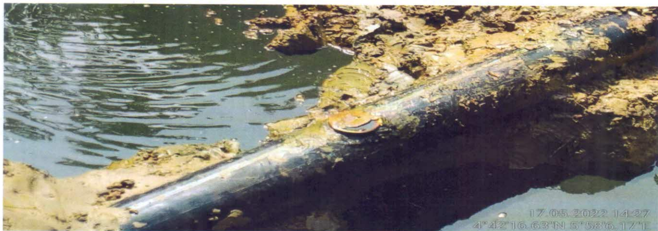
DISCONNECTION OF INSTALLED VALVE POINT SHOWN
